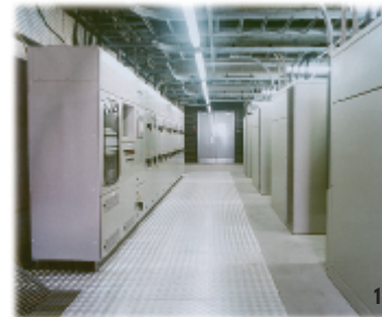
Fixed Ground Power Room 5 x 315 KVA incl. 400 Hz distribution
