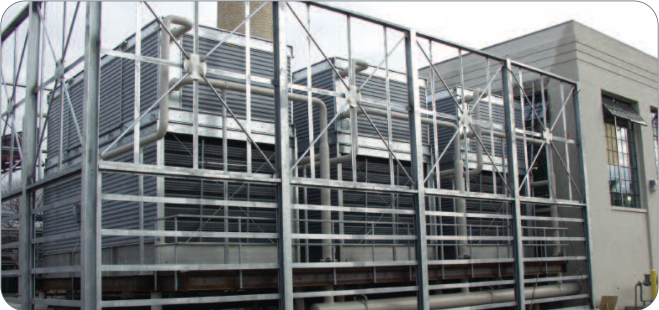
Figure 10 - Architectural Walls Being Constructed Around FXV Closed Circuit Cooling Towers
