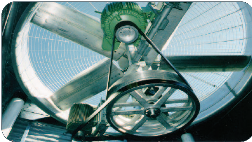
Figure 6 - BAC Axial Fan Cooling Tower Utilizing the BALTIGUARD™ Fan System
