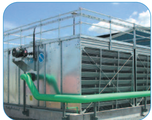
Gear Drive System, Externally Mounted Motor
