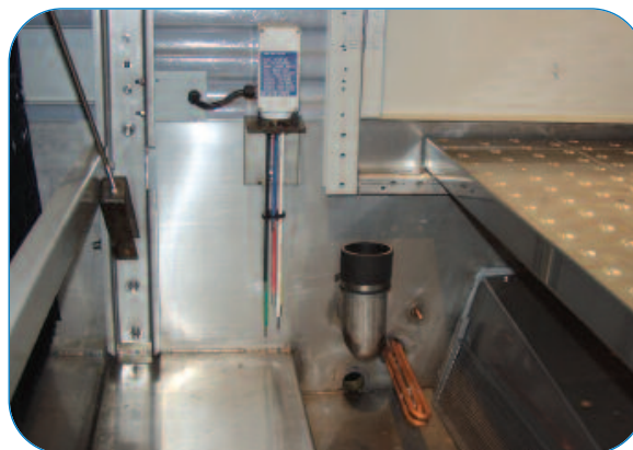
Electric water level control package and basin heater
