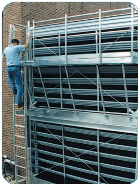
External Platform at Louver Face
