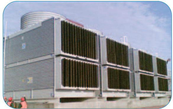
Unit With Intake Sound Attenuation
