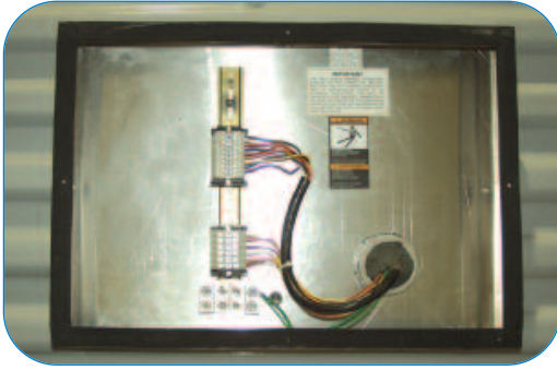
Externally Mounted Terminal Box
