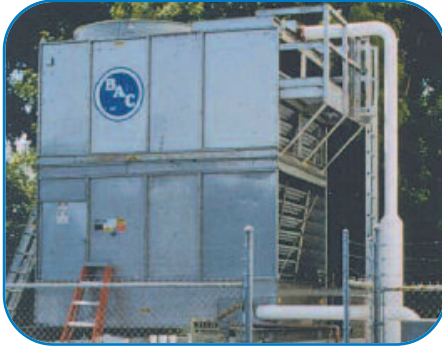
Series 1500 with Optional External Service Platform
