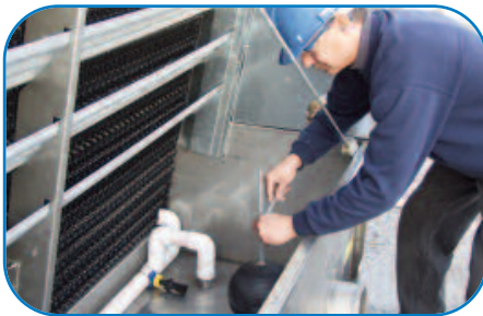
Access to Strainer, Make-up and Basin Accessories from Outside the Tower
