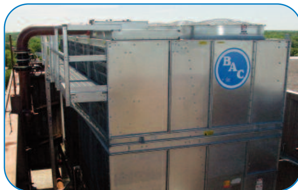
Single Side Air Inlet Provides Installation Flexibility in Tight Layouts
