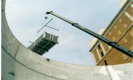
Ice Coil Pattern Inside Steel Tank
