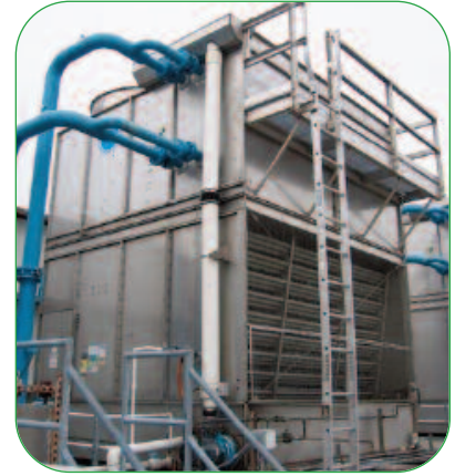
External Platform at Louver Face
