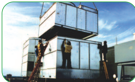
The Unit Shown Ships in Two Pieces to Minimize Shipping and Rigging Costs
