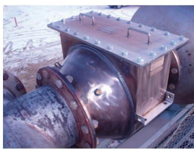
DCL International has developed the next generation of its QUICK-LID catalytic converter systems for stationary diesel and natural gas engines. The newest units incorporate features designed to improve serviceability and access.
