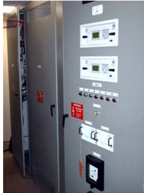
Figure 9. Cabinet with Redundant Digital Excitation Control Systems
