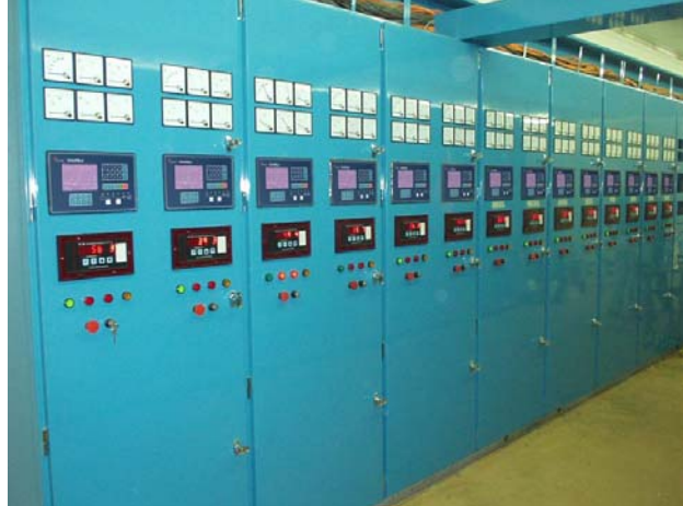
Engine control panels
