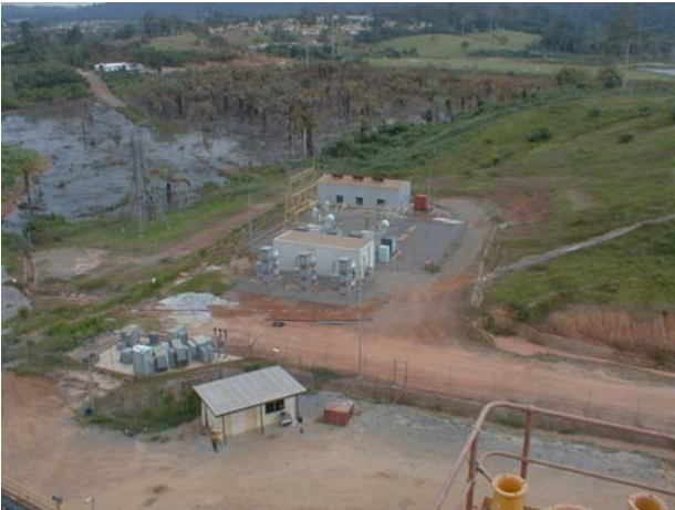
HV substation with 2x33kV line incomers
