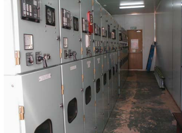
Circuit breakers for 11kV in HV substation
