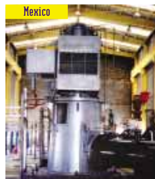
Mexico Four City Municipality Water Pumps at 4160V / 400A elevating Fresh water to 1800 Meters
