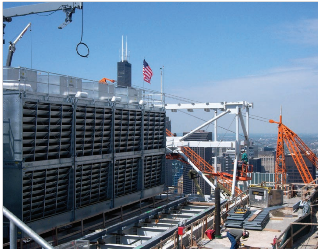
F.E. Moran partnered with Baltimore Aircoil Company on a cooling solution to accommodate a two-stage construction process. Cooling towers were designed to fit into tight spaces and to be easily removable upon completion of the building.
