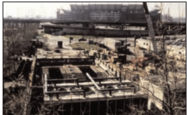
PSINet Football Stadium (Ravens), Baltimore MD Ice Thermal Storage 13,600 Ton Hours (47,818 kWh) 1,132,880 lbs. of ice (513,874 kg) also Cooling Towers
