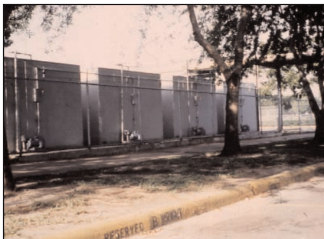
Lee College, Baytown TX Ice Thermal Storage 5,535 Ton Hours (19,461 kWh) 461,065 lbs. of ice (209,139 kg)
