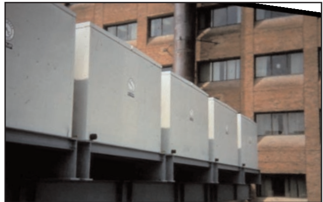
Union Memorial Hospital, Baltimore MD Ice Thermal Storage 7,210 Ton Hours (25,315 kWh) 599,760 lbs. of ice (272,051 kg)
