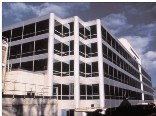
Johns Hopkins Applied Physics Lab, Laurel MD Ice Thermal Storage 22,400 Ton Hours (78,758 kWh) 1,865,920 lbs. of ice (846,381 kg) also Cooling Towers
