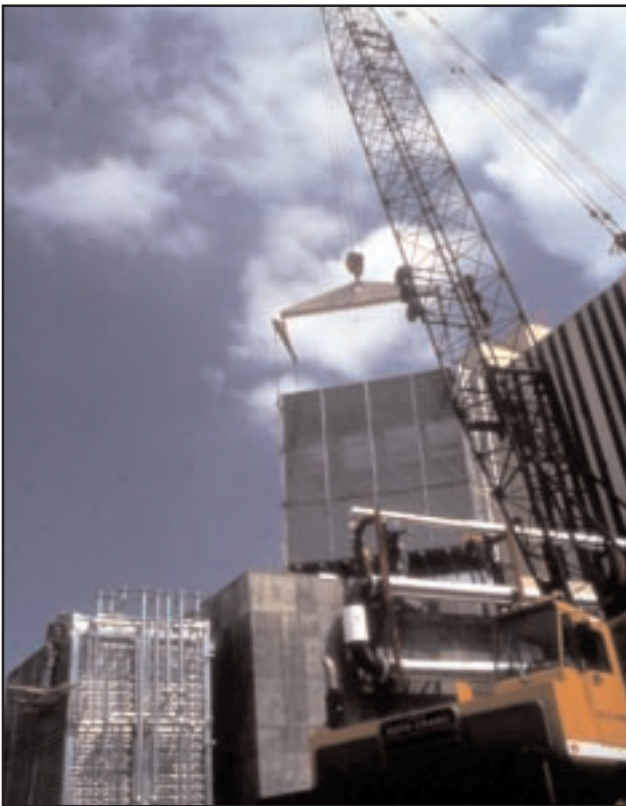
John Peter Smith Hospital, Fort Worth TX Ice Thermal Storage 14,800 Ton Hours (52,037 kWh) 1,232,840 lbs. of ice (559,216 kg) also Heat Exchangers and Cooling Towers
